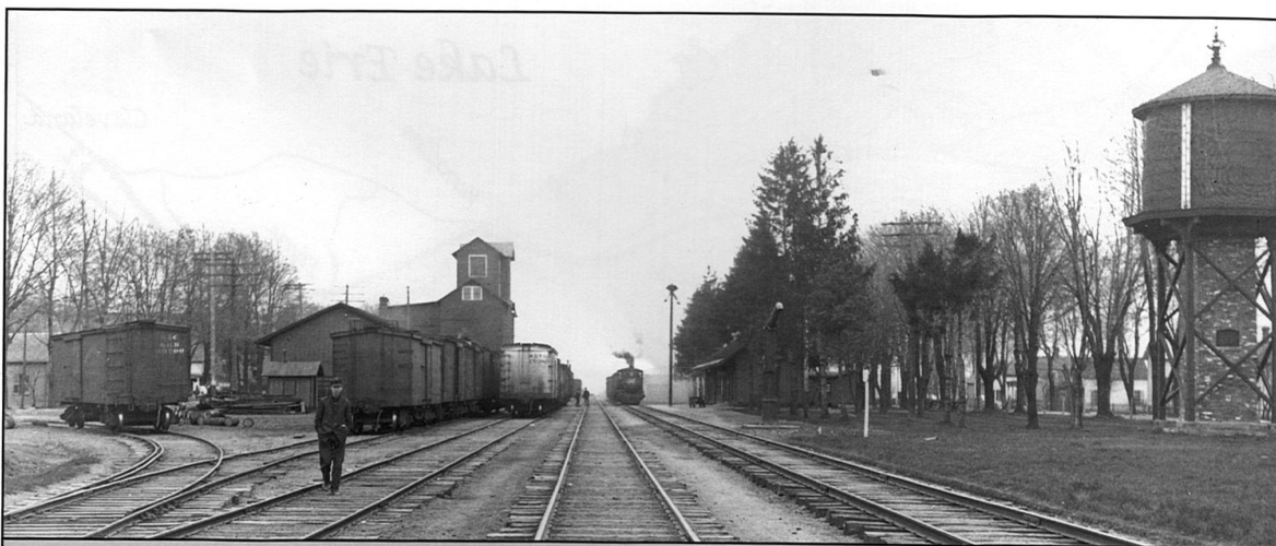
On a bleak winter day in 1900, a westbound train approaches the depot at Elmore on the original TN&C track, the "Norwalk Branch" of the NYC. Built as a single track line, it remained so for its entire existence. This scene is typical of most of the towns and small cities along the way. In each town there would be a depot, a few sidings to service the local elevator and other small businesses, and a water tank and coal yard for the locomotives. The water tower on the right, deemed an eyesore by local residents, was removed in the following year. Photo courtesy of the Grace Luebke Local History & Genealogy Department, Harris-Elmore Public Library.
