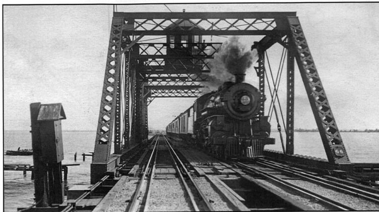
LS&MS K-2d 4806, built by Alco-Schenectady in July of 1907, rolls over the Sandusky Bay Bridge around 1910. Curiously, the 45 LS&MS Pacifics in subclasses K-2a through K-2d, built between May and July of 1907, were numbered in reverse order, with K-2a 4844 delivered first, and K-2d 4800 delivered last. Photo by Ernst Niebergall. Charles E. Frohman Collection/Hayes Presidential Center.
