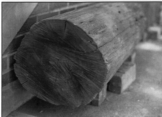
Here is an actual segment from one of the Ohio Railroad pilings. Roughly a foot in diameter, this particular specimen is in very good condition for being over 110 years old when photographed in 1957. Charles E. Frohman Collection/Hayes Presidential Center.
