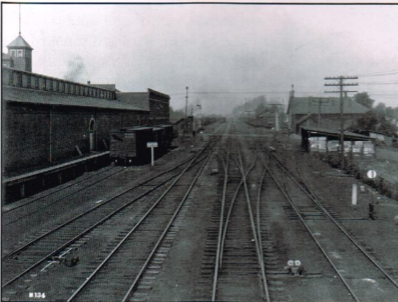
This view looks west along the three-track bypass from the American Crayon Company building, on the left. NYCSHS Archive Image PB505.043.
