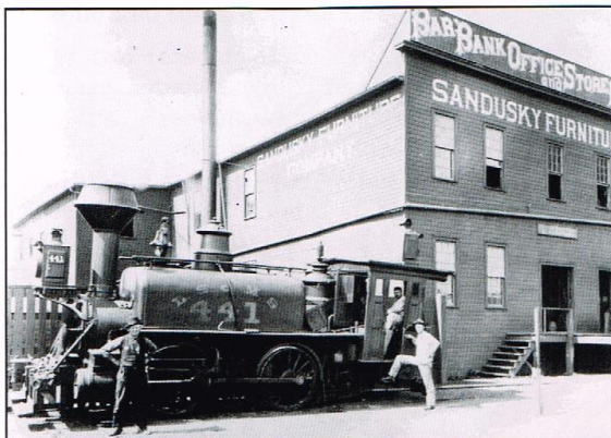
LS&MS 441, a home-built, four-wheel tank engine dating back to 1872, was switching at Sandusky sometime before her scrapping in 1895. Climbing into this locomotive's commodious cab did not require much effort. Ray Curl Collection, NYCSHS Archive Image PB626.145.
