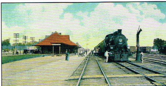
In this colorized, early 1900s postcard view, a Toledo-bound passenger train pauses at Sandusky. While mail and express is loaded and unloaded, the engineer takes care of his steed's needs. The power is one of the LS&MS's high-stepping 2-6-2 Prairies. Collection of the author.
