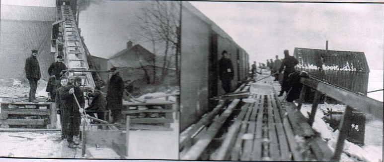
This quintet of photos depicts five of the several processes that brought considerable revenue to Vanderbilt coffers from Sandusky's ice-harvesting business. They demonstrate using a horse-drawn steel scoring device to mark out the blocks of ice, sawing the blocks, floating the blocks in a channel to the ice house (note the wintering Cedar Point steamers), feeding the blocks into an ice house, and loading the blocks into a boxcar. Sandusky Public Library.
