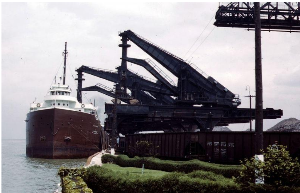
Hulettts at work in Cleveland Photographed for the Farm Security Administration, May 1943
